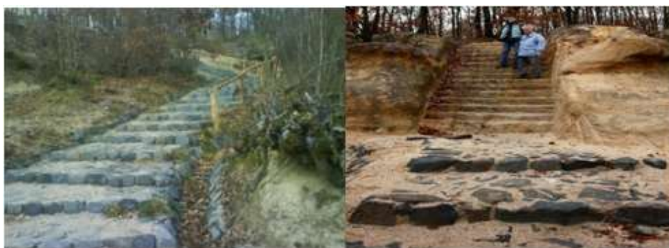
Fig. 30. Realization of successive stairs, photo Aurica Grec, 2015
