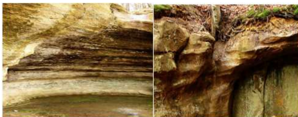
Fig. 28. Figure 2. Mining gallery, photo Aurica Grec, 2015
